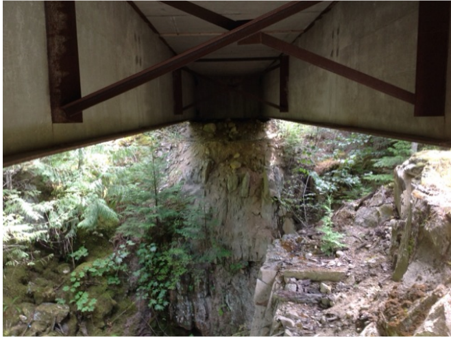
Left Bank Abutment when facing downstream
