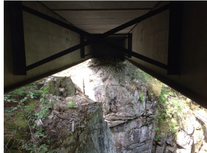
Right Bank Abutment when facing downstream
