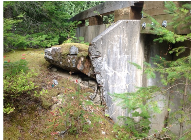
right downstream ballast wall
